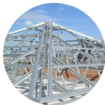
Steel bar truss
